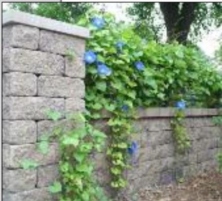
To make strong connections with the wall panel and post/pillar, extend the top course of wall panel into the post/pillar using a Corner Block. If building a wall panel taller than 5 courses, we recommend interlocking it into the post/pillar to help stabilize the wall.
