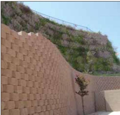
The south walls were cut walls with maximum heights of 50 ft (15.2 m) and the north walls were fill walls with maximum heights of 25 ft (7.6 m). Obviously, the design of the retaining walls required involvement from all engineering parties contracted for the project. There were many design factors that
