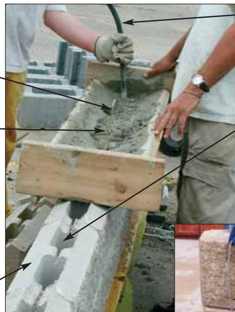
Small diameter stinger vibrator to assist the flow of grout around rebar.
